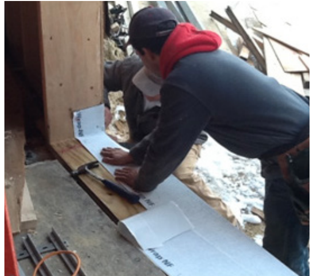
Flexible Sill Pan Installation
