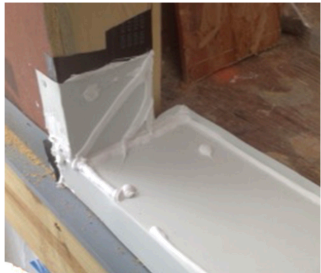
Rigid Sill Pan Installation
