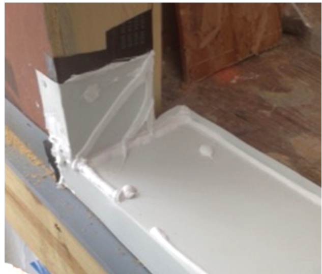
Rigid Sill Pan Installation
